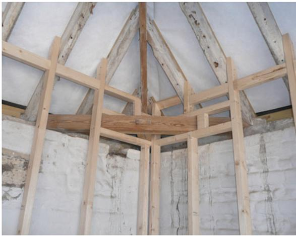
slightly off the wall to allow the foam to get behind the studwork to provide a weatherproof seal against driving rain and rising damp. A perfect air tight seal between the walls and the roofs of the barns is created in a seamless coating of foam. Any fungal growth on the wall surface is prevented and the foam eliminates any space for insects or rodents.
